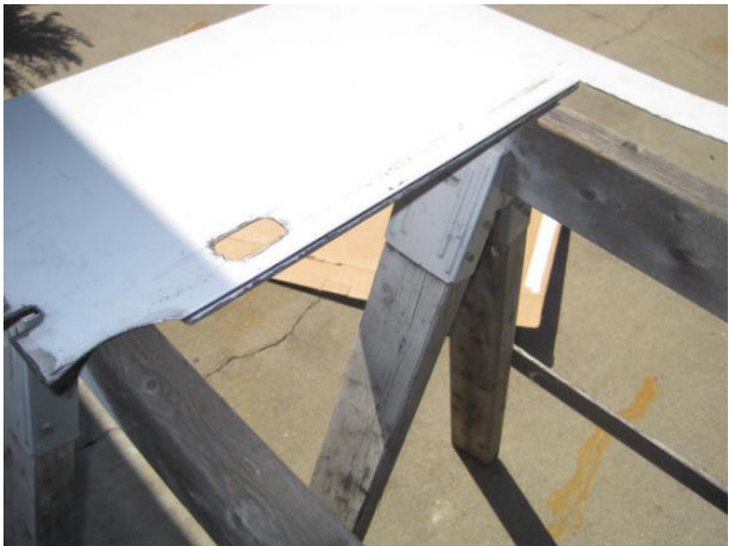
Bending the lip at the hatch opening - old school technique.
