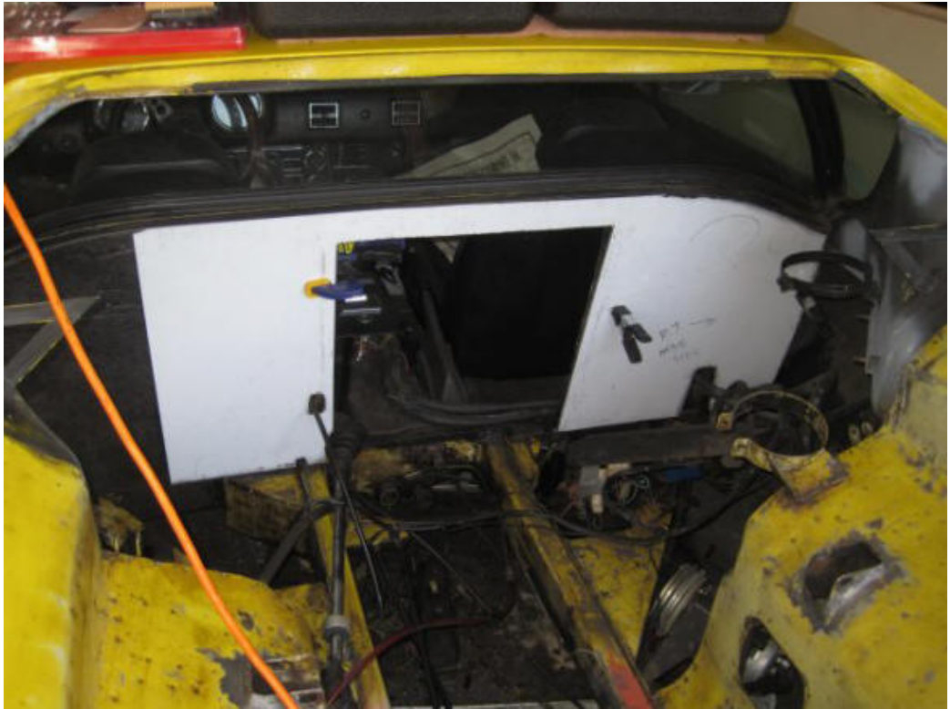
Firewall Reduction Kit from Kirk Evans Welded up the bulkhead reduction hatch cover.
