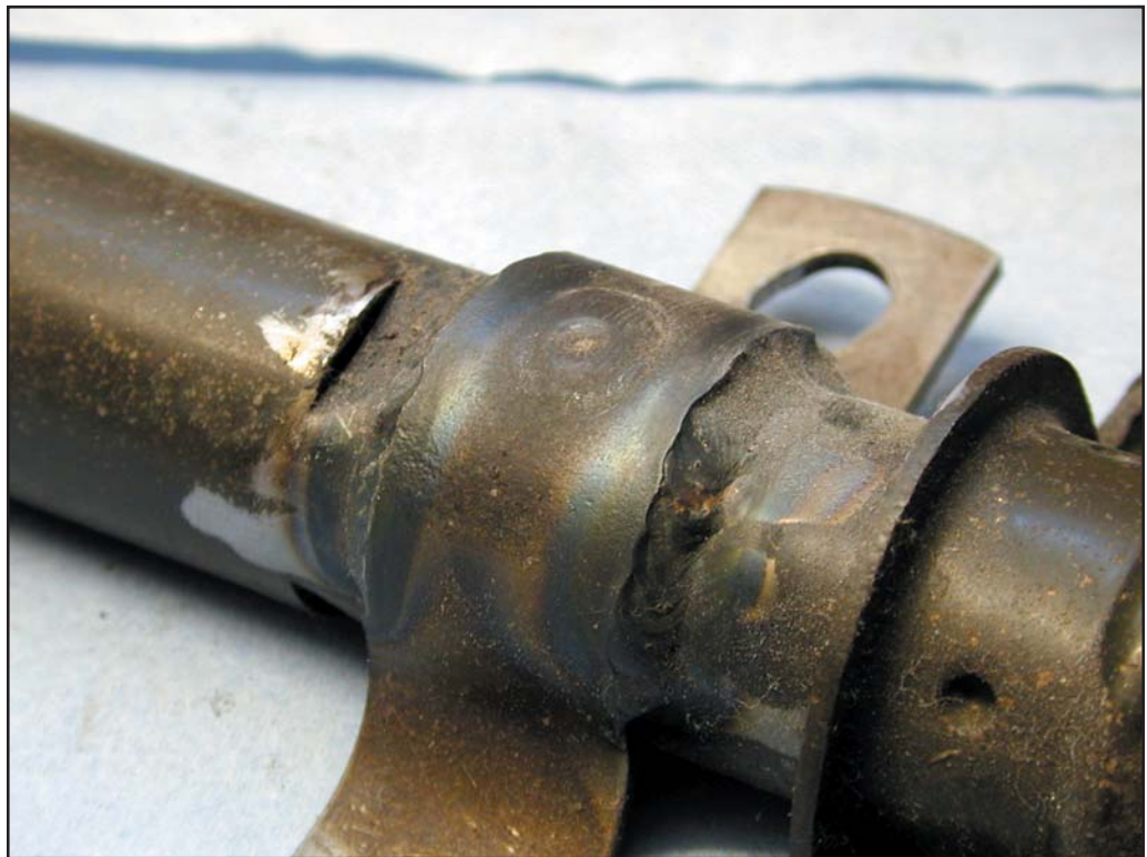
The mounting bracket for the steering column tube is held in place with just a single spot-weld in the center of the bracket; on this car, as most cars, this weld was broken. This bracket was seam-welded along its entire length. Note the indentations on the left which locate the bottom bearing. Be sure to fully remove the remnants of the nylon bushing before welding the bracket, or the heat will melt the nearby bushing and make a real mess. (Don't ask me how I know this!)
